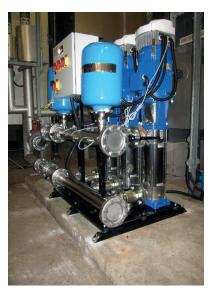
Booster pump pressure vessels are essential components in any system that relies on steady and consistent water pressure. They help to reduce pump wear, improve energy efficiency and ensure reliable water supply.
