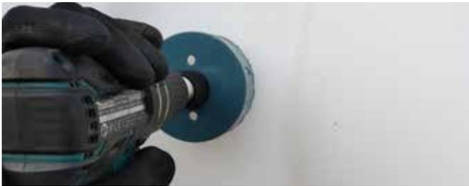
Drill 140mm for 110mm diameter pipe with whole saw and clean off burr.
