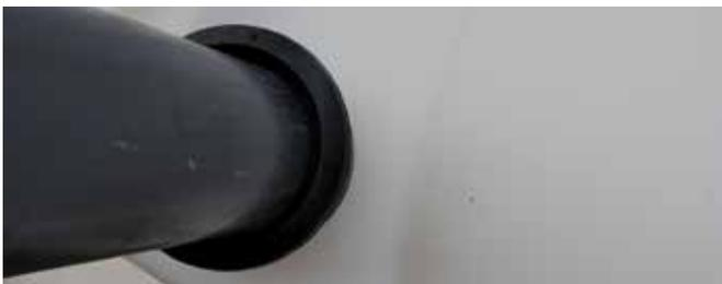
Once the wall seal is in place the pipe can be inserted into the seal. The seal can be sprayed with soapy water to ease pipe installation.
